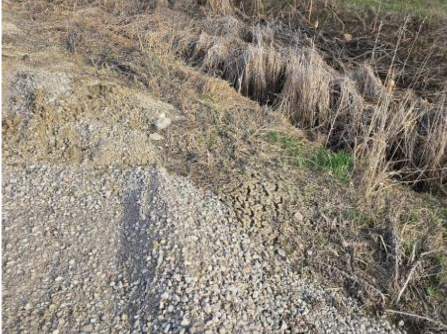
SOUTH SIDE OF PROPERTY FACING SOUTH
