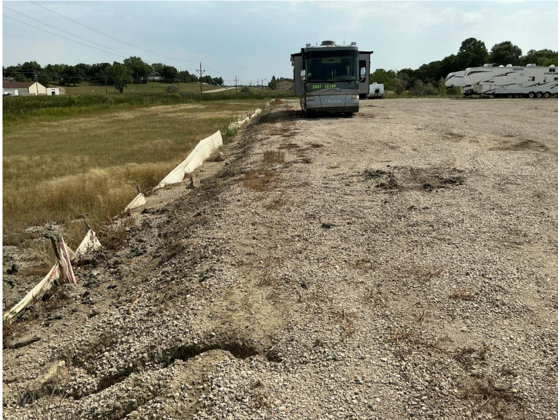
View from north side of “developed” property facing east, slightly west of NoDak Recreation trailer parked at NW corner of entrance/exit of property.
