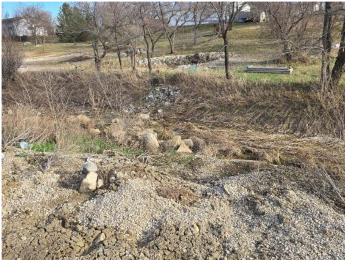
SOUTH SIDE OF PROPERTY FACING SOUTH
