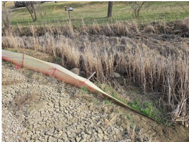
SOUTH SIDE OF PROPERTY CLOSEST TO 52ND ST NE FACING SOUTH
