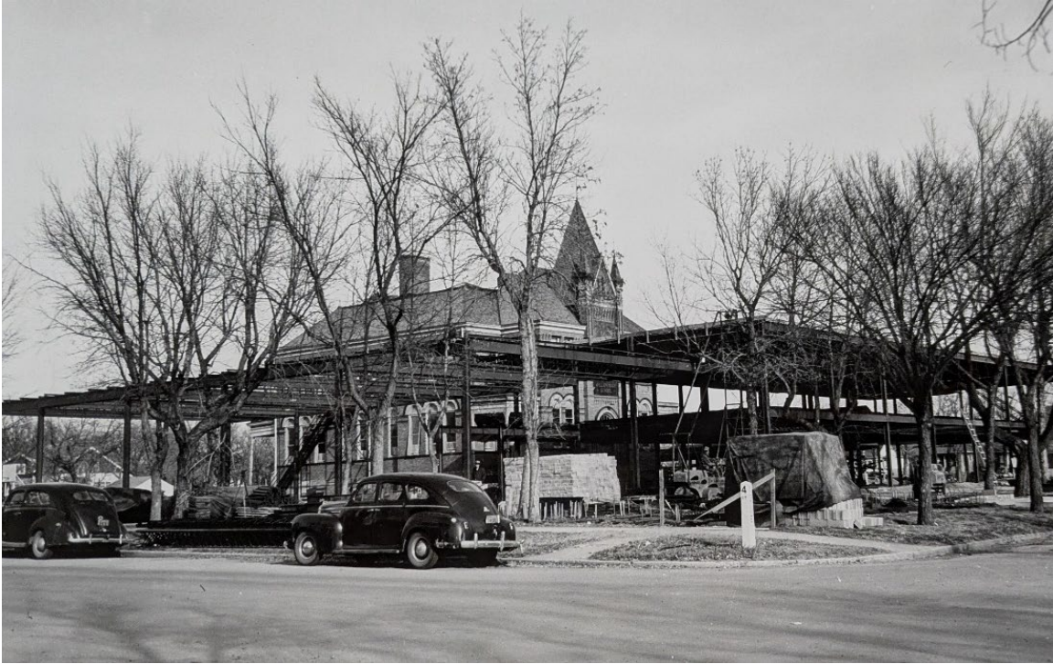
Figure 17: Will-Moore Elementary School under construction, with the previous school building visible in the background. Photograph by Leo LaLonde, c. 1950. Courtesy of Will-Moore Elementary School.
