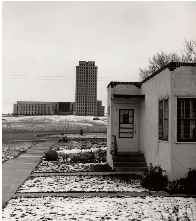
Figure 16: View looking up fourth Street towards the relatively new North Dakota State Capitol building, 1940. Photo depicts the entryway of 1023 N 6th Street in the foreground, which was completed that year. John Vachon Photograph Collection, item ND 11-1940, State Historical Society of North Dakota.
