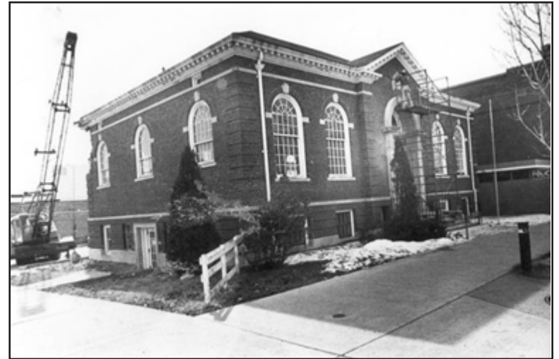
Preparing for demolition of the former Carnegie Bismarck Public Library, located at 6th Street and Thayer Avenue, in 1980. Image courtesy of Bismarck Veterans Memorial Public Library (Bismarck: Capital City Memories 1c-30).
