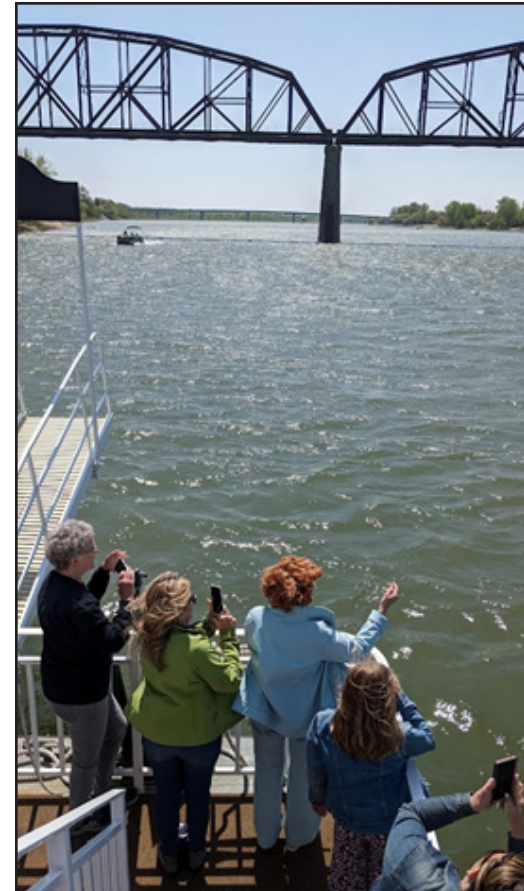
Passengers aboard the Lewis & Clark Riverboat take photographs as they approach the 1883 Northern Pacific Rail Bridge spanning the Missouri River. Photo courtesy of Friends of the Rail Bridge.
