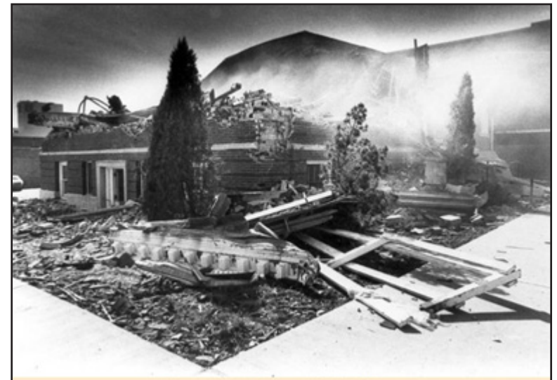
Ruins of the former Carnegie Bismarck Public Library, demolished in 1980. Image courtesy of Bismarck Veterans Memorial Public Library (Bismarck: Capital City Memories 1c-33).
