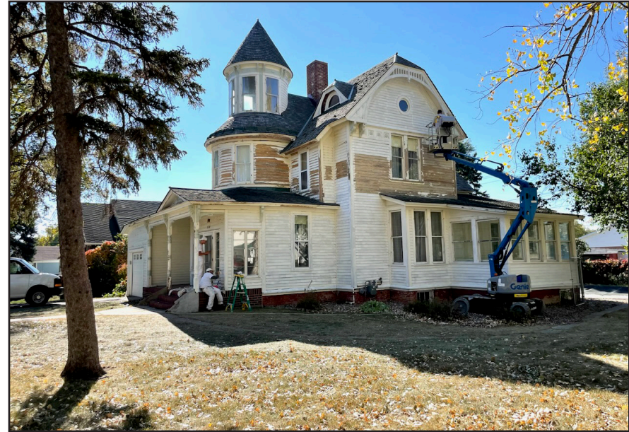
Workers scrape paint on the exterior of the 1883 Dr. Porter House (824 N 4th Street) during a recent restoration project. Photo by Tom Stromme.
