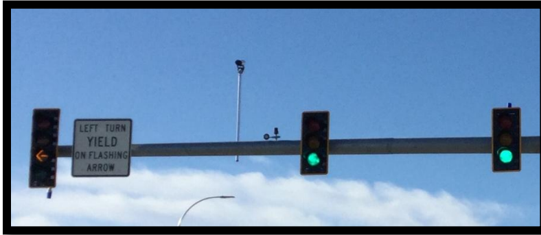
Figure 6 Video and Optical Detector for Preemption
