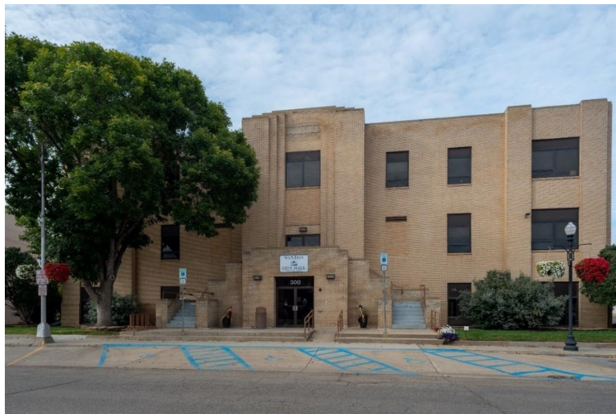
Figure 3 Mandan City Hall (Engineering Department)
