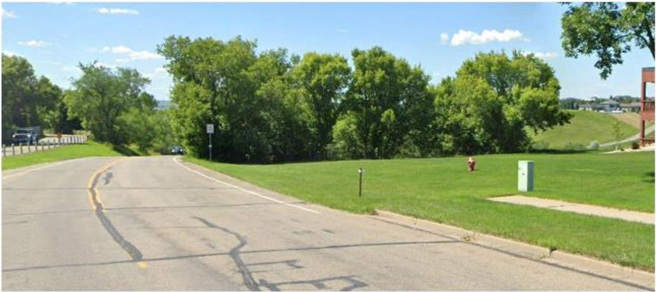
Figure 2 Burnt Boat Road end of sidewalk
