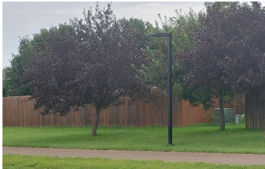
Figure 4 – Example Lighting Structures
