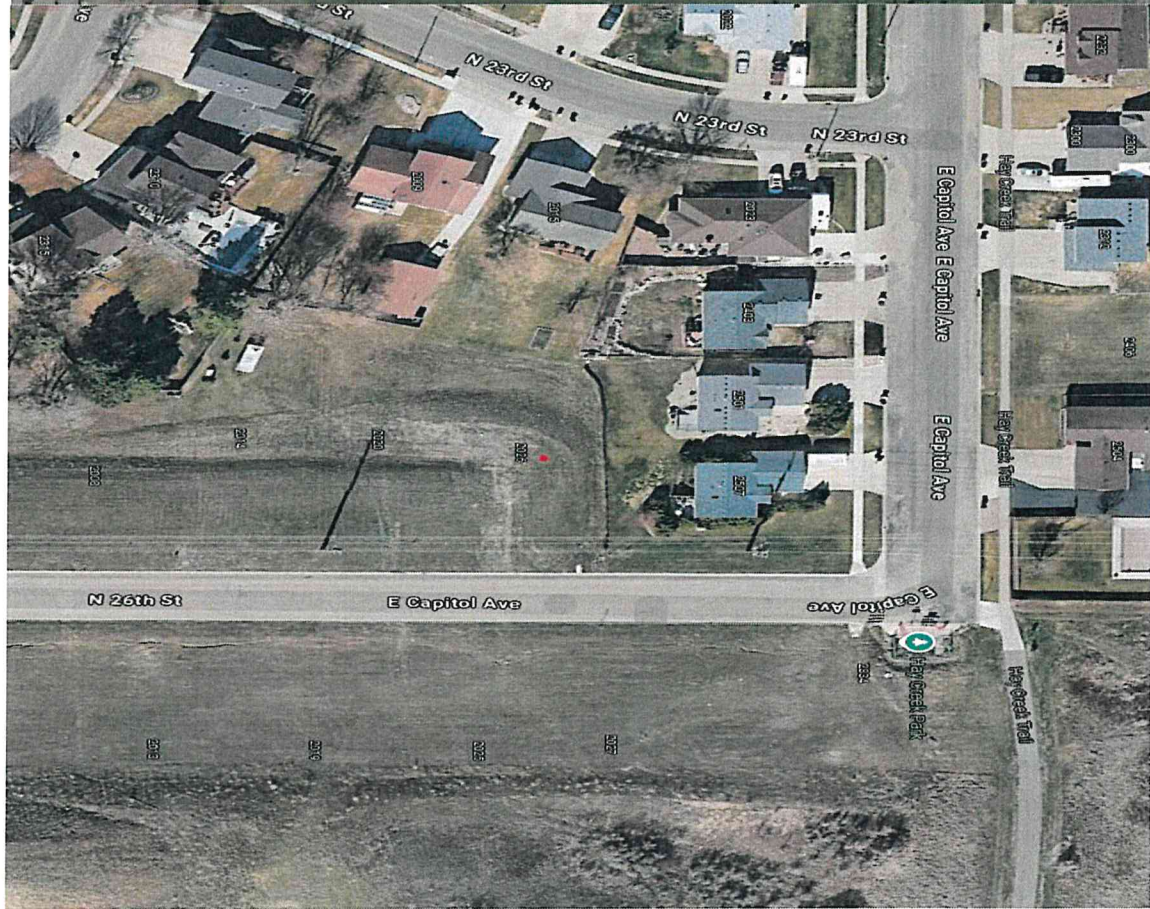
After 26 th Street Construction. Drainage Lot
