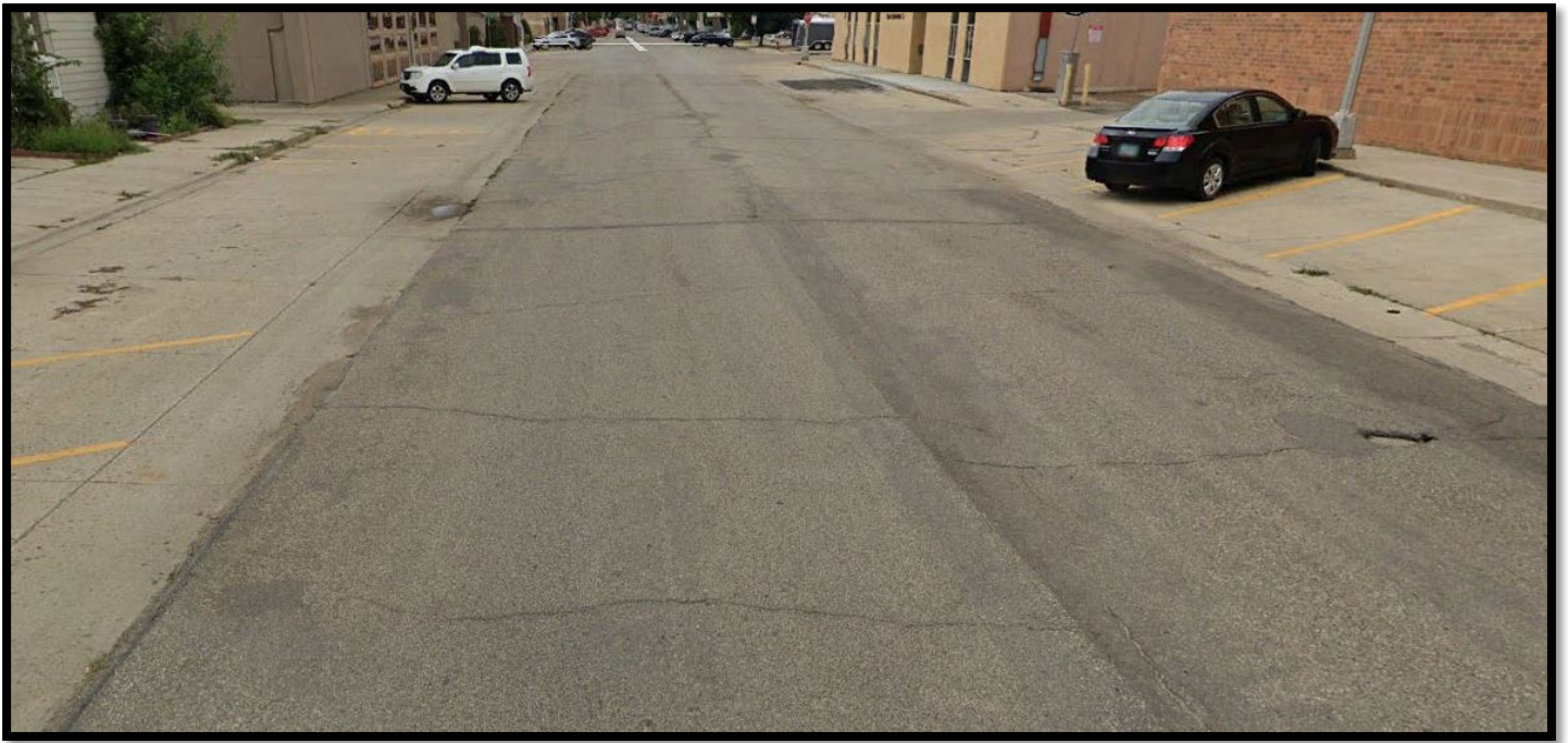
1 st Street NW between 4 th and 5 th Avenue looking east to 4 th Avenue above
