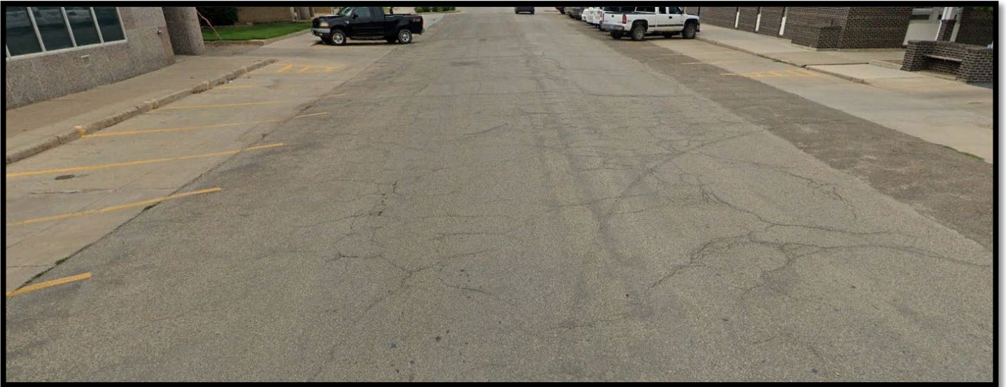
1 st Street NW between 2 nd and 3 rd Avenue looking east to 2 nd Avenue above
