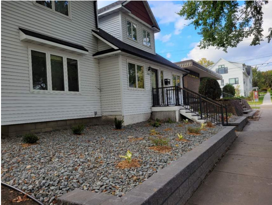
Existing Condition of 418 North 2 nd Street
