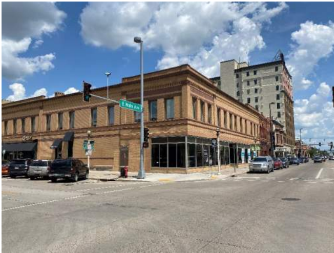
Existing Conditions of 402 East Main Avenue
