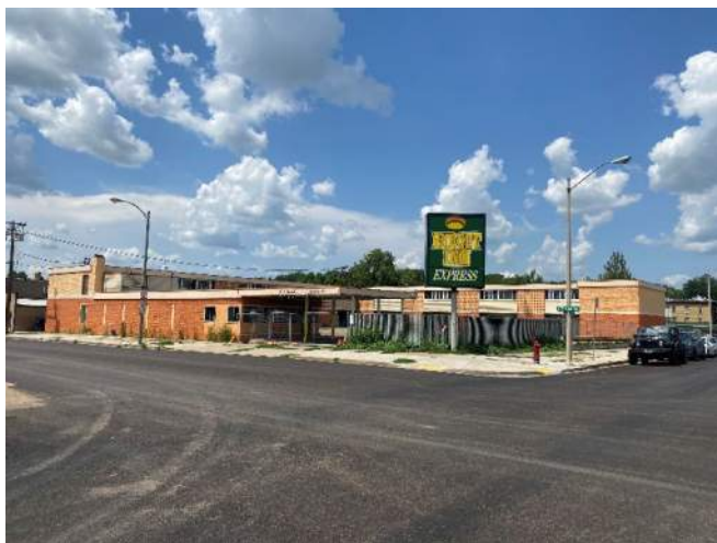
Existing conditions of 122 East Thayer
