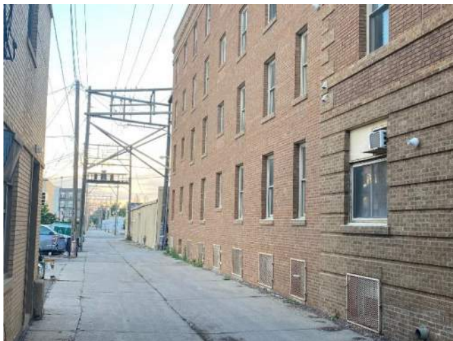
South Wall of 114 N 3 rd Street
