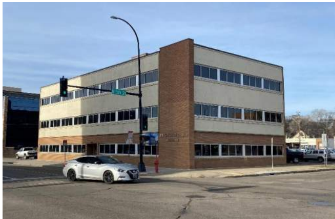
Current Condition of Building at 418 East Rosser Ave
