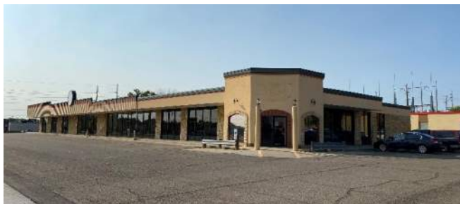
Strip mall proposed for demolition
