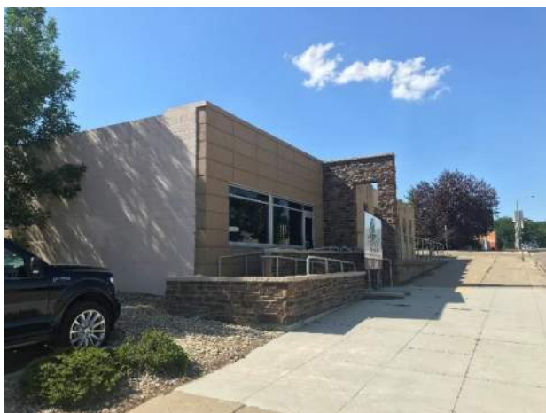
Front of building from N 2 nd Street
