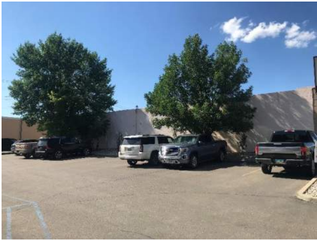
South side of building where windows planned
