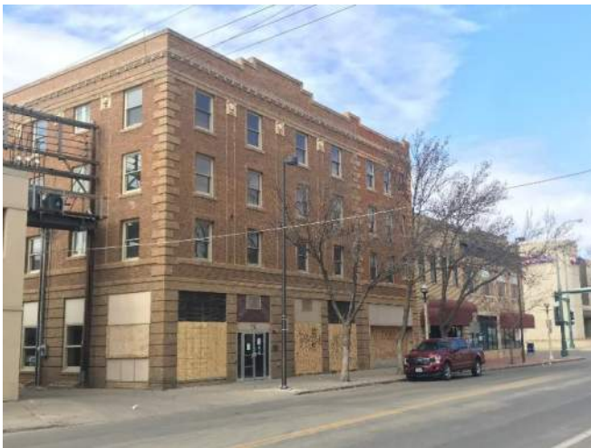
Existing Condition of 114 N 3 rd Street
