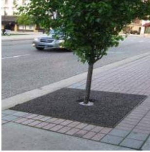
Example of flexible porous pavement
