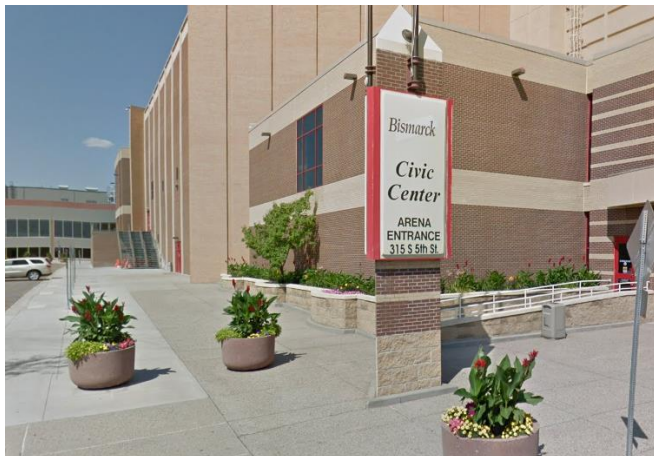
Existing monument sign proposed for alteration
