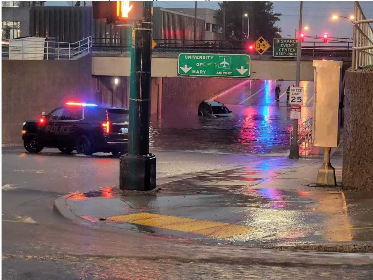
Exhibit B: 7 th Street Underpass looking south during storm event
