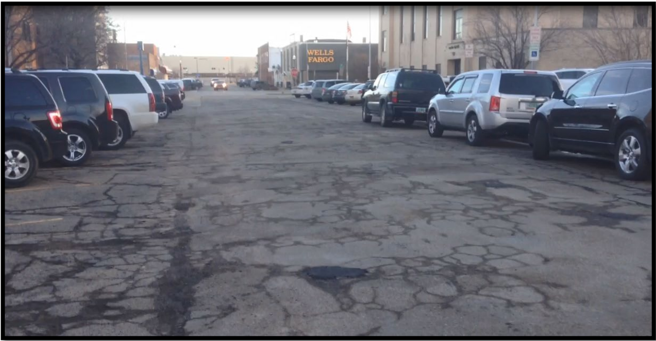
2 nd Avenue NW between 1 st and 2 nd Street looking south to 1 st Street above (December 2017)
