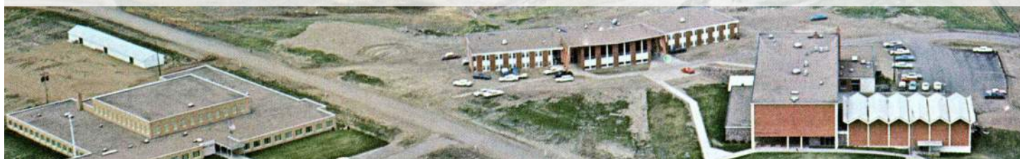
Aerial view of Bismarck State College viewed from south. Courtesy of Bismarck State College.
