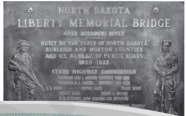
Above: Detail of dedication plaque of the Liberty Memorial Bridge. Historic American Engineering Record HAER ND,8-BISMA,2- (Library of Congress). Below: Postcard of the Liberty Memorial Bridge. Courtesy of Jason Tomanek.
