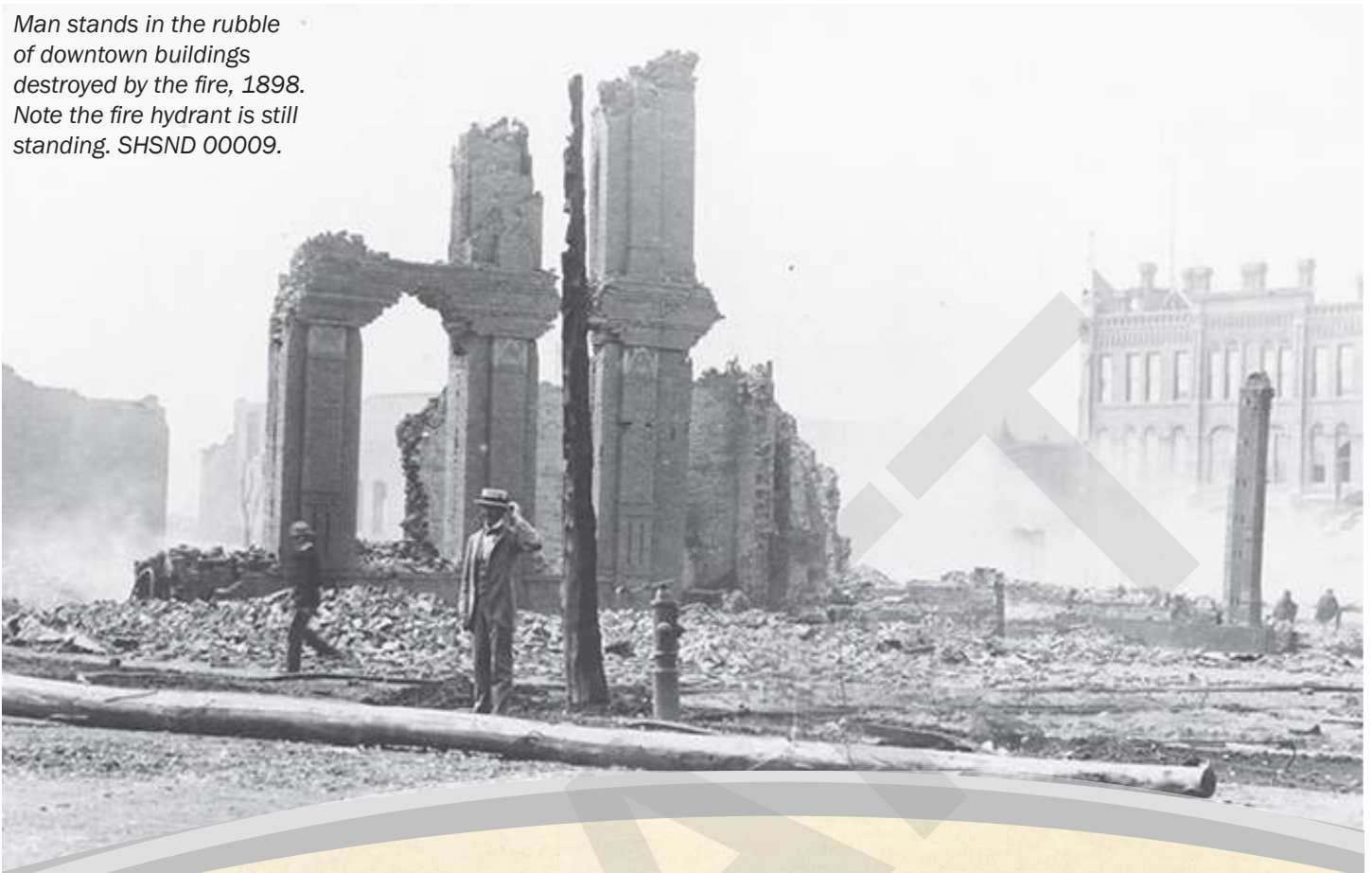
View northeast across Main Street depicting the aftermath of the 1898 fire. SHSND 00111-02.
