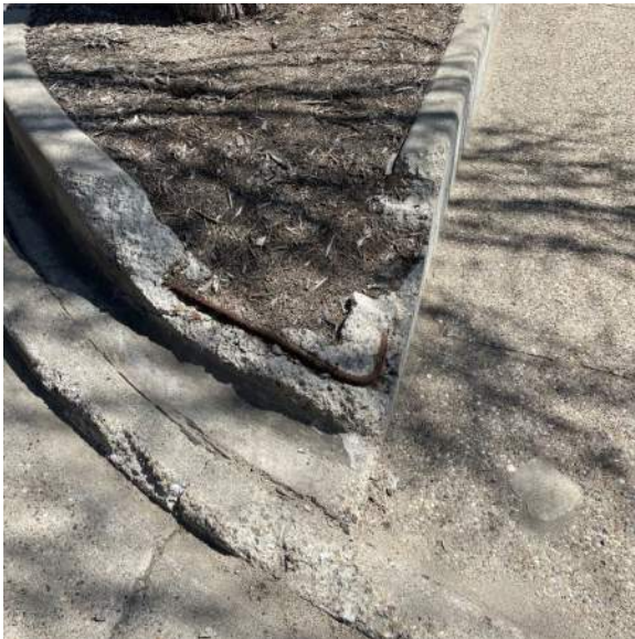
Missing concrete on corner of a raised planter – structural rebar exposed
