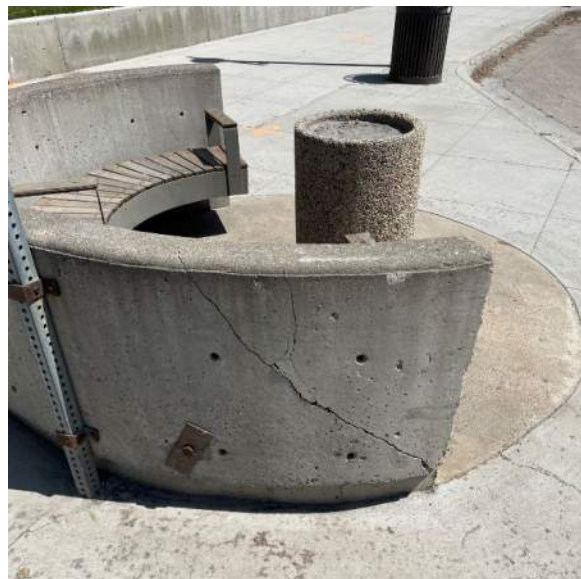
Missing concrete on corner of a raised planter
