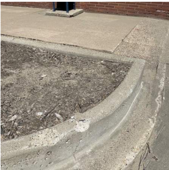
Missing concrete on corner of a raised planter – structural rebar exposed
