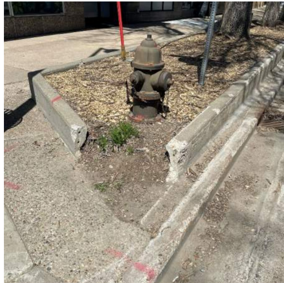
Missing concrete on corner of a raised planter
