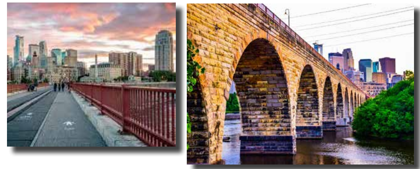
[figure 6.2 & 6.3] stone arch bridge minneapolis, minnesota
