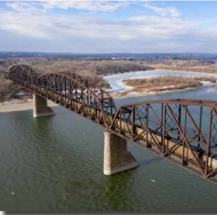
figure 1.0] aerial drone view of high bridge
