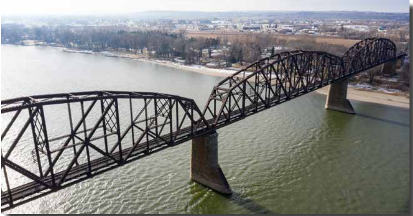
[figure 1.1] aerial drone view of high bridge
